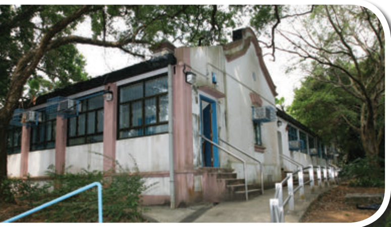
舊大埔警署 (23)* Old Tai Po Police Station
